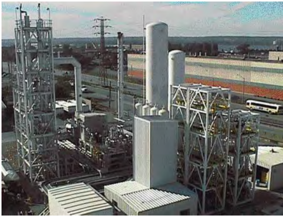
Figure 2.7. Atomic Energy of Canada Ltd. advanced heavy water pilot plant, Hamilton, ON. Photo courtesy Atomic Energy of Canada Ltd. This plant produced about 1 ton of heavy water per year. A scaled up version of it would be more efficient and cleaner than the old Bruce Point plant, shown above.
