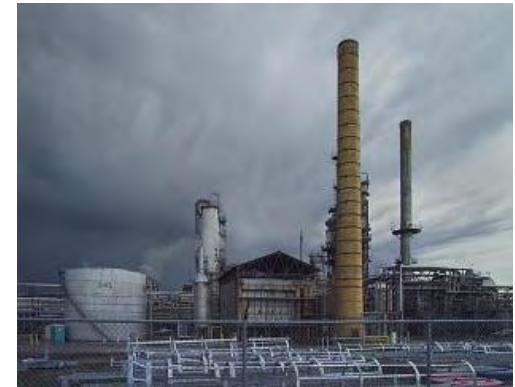
Coal Power Plant
